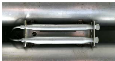
Typical high-limit/sensor probe locations and mounting hardware.
